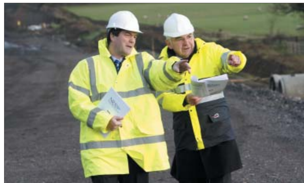
Last 25th January, Minister of Transport T.D. Mr. Noel Dempsey visited the M3 Clonee to North of Kells project. Mr. Peter Malone, Chairman of the National Roads Authority was explaining to him the good progress of the works.
